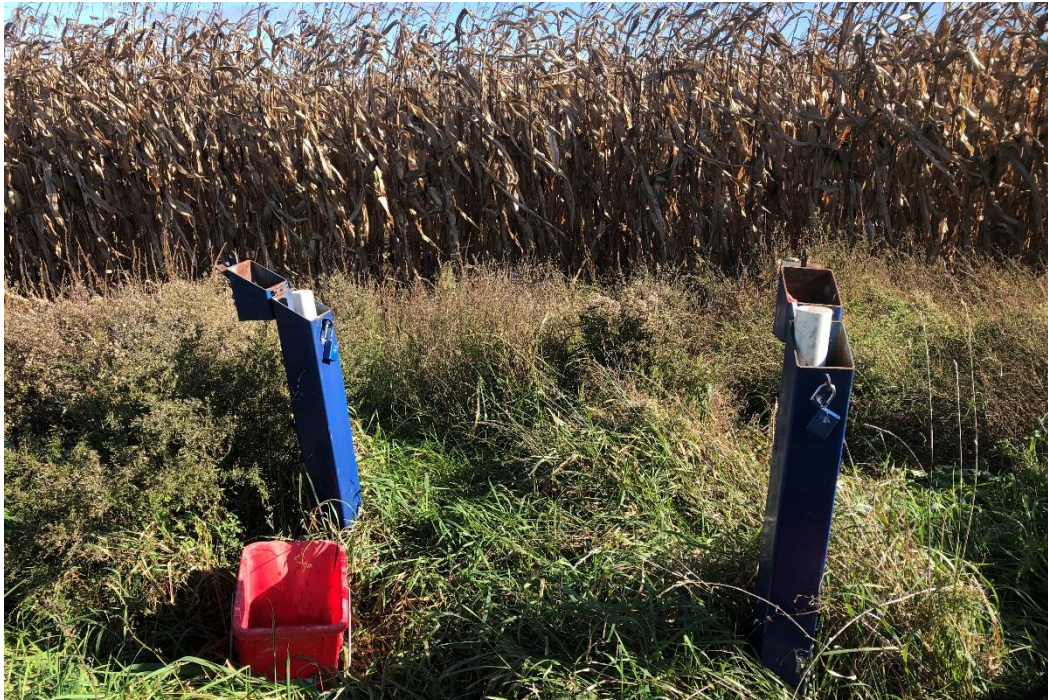
Photo 17: View of monitoring well MW102 and MW103 looking southeast (October 2021).
