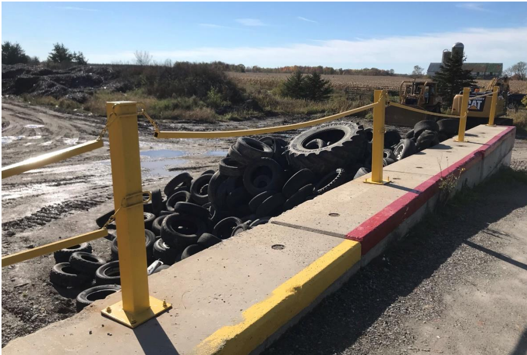
Photo 3: View of tire storage next to the transfer facility (October 2021).
