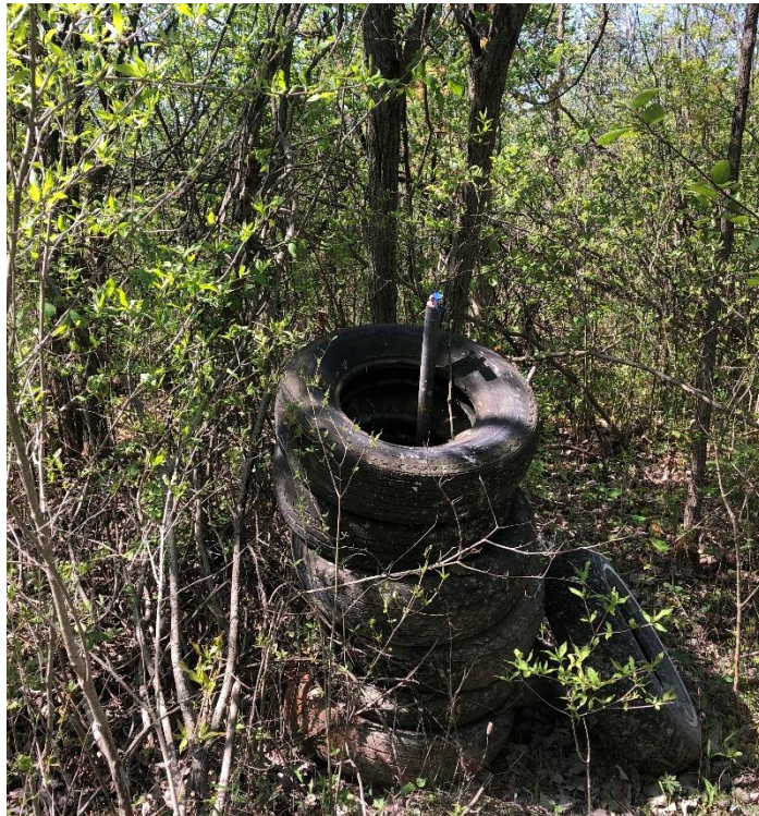
Photo 16: View of monitoring well 91-3 looking southwest (May 2021).
