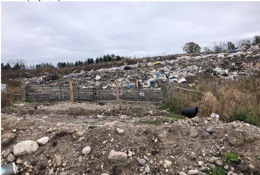
Photo 2: View of the gate with new deterrent trench, at the front west side of waste face (October 2021).
