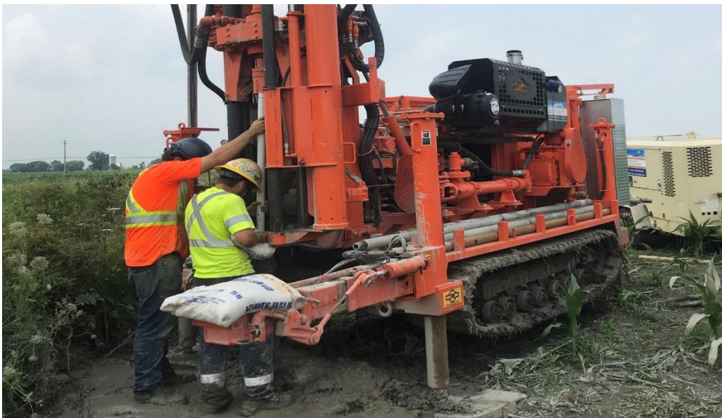
Photo 20: Installation of MW301 looking north (July 2021)
