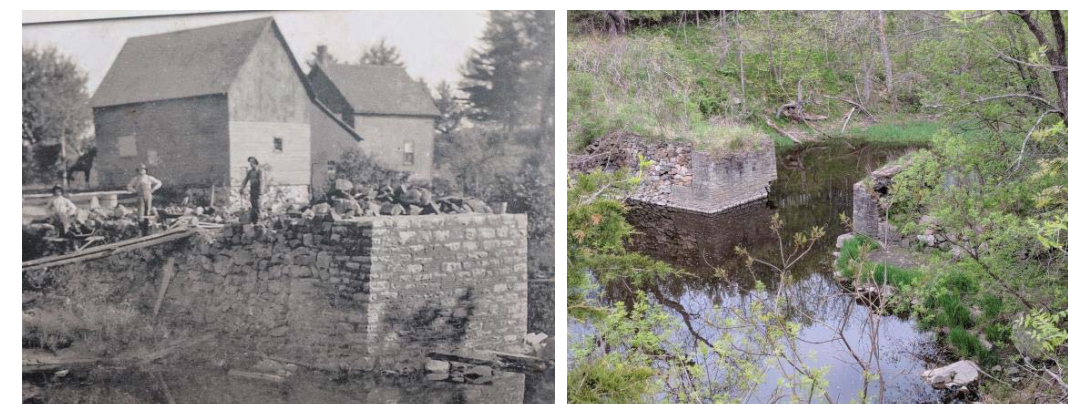
LTI-17 Early Photo of Crossing
