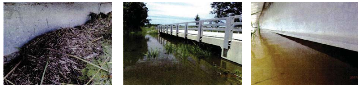
LTI-1 Debris caught up at east girder LTI-1 West elevation LTI-1 Sag in west exterior girder
