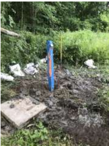
Photo 19: monitoring well OW24R01 following installation (July 2021)
