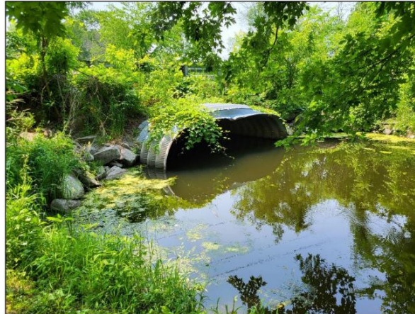
North elevation (deformation at culvert obvert)
