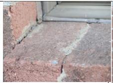
Mortar and sealants are failing around windows. This needs to be addressed to avoid water penetration and freeze thaw damage.
