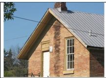
Soaked brick the result of failed flashing at the chimney, neds to be repaired aling with general roof repairs.
