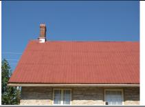
Metal roof in fair condition with eave repairs required
