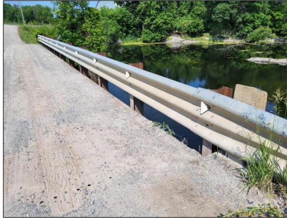
North Barrier (Thrie Beam)
