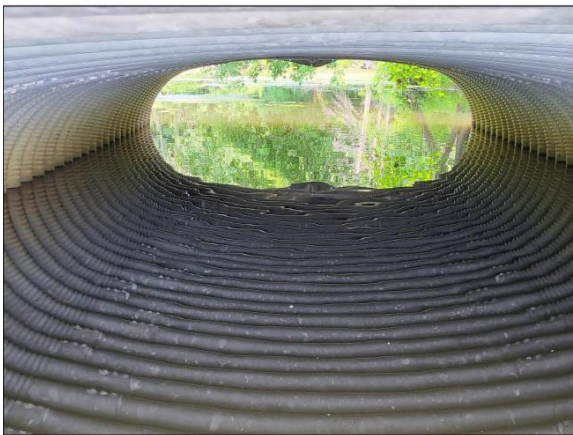
Looking north through barrel
