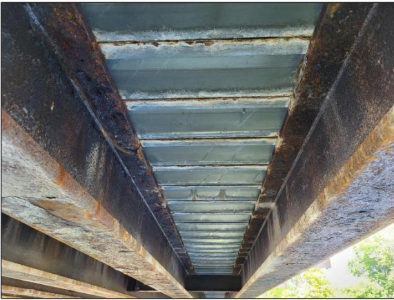
Deck Soffit & Girders
