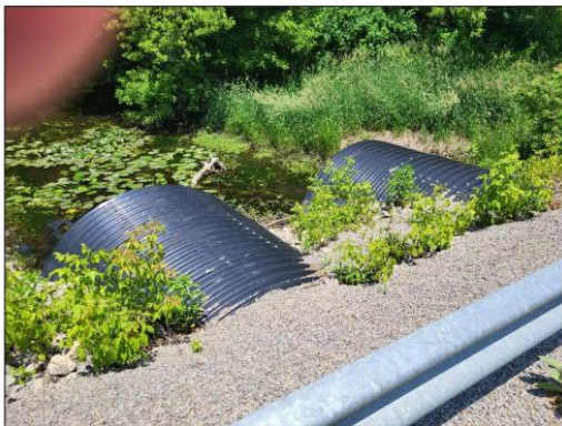
Barrel Ends looking north
