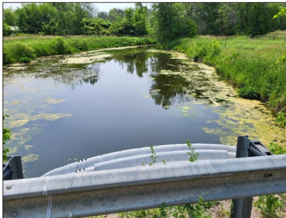
Barrel outlet (downstream)
