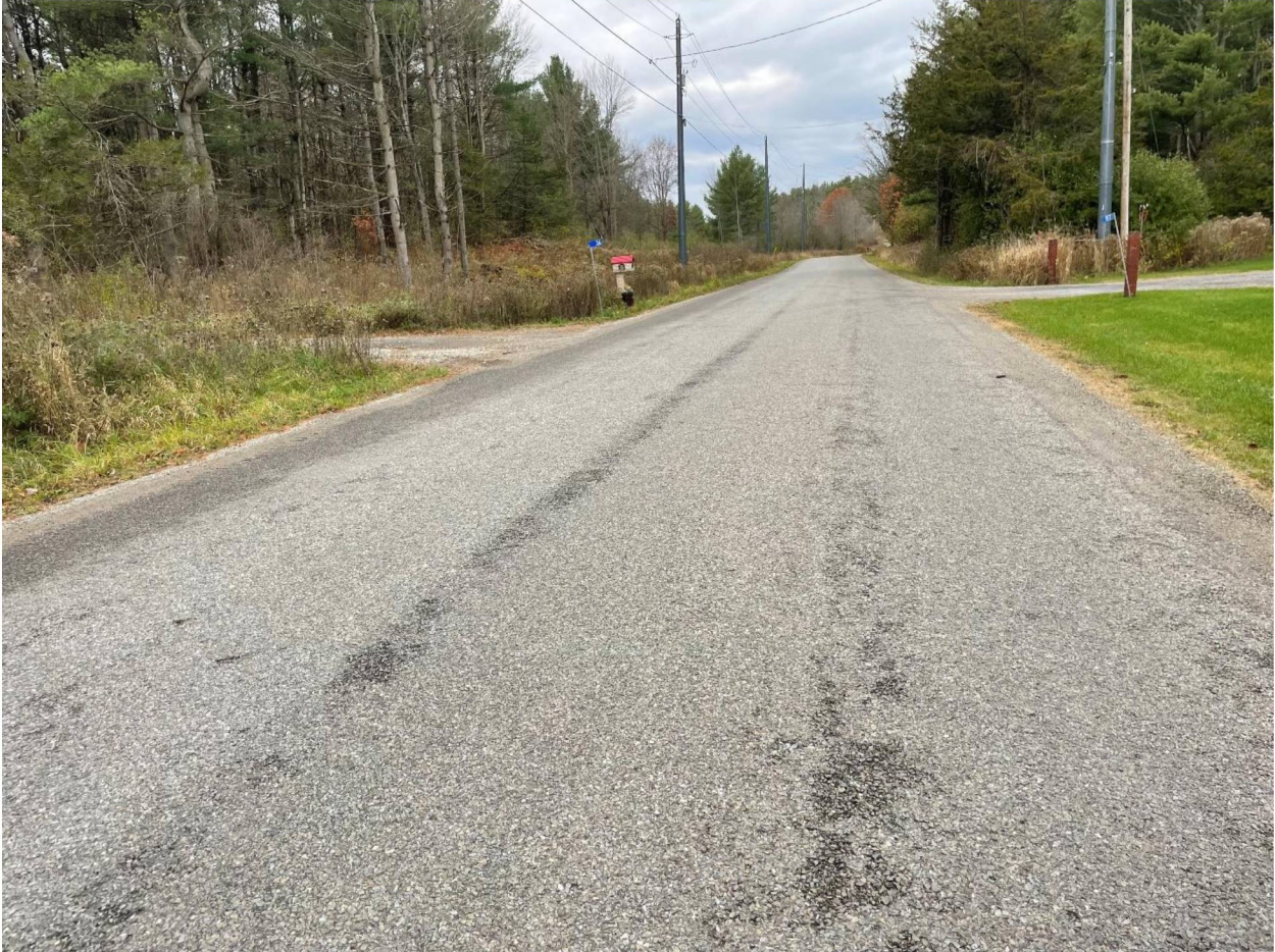
Figure A2 – Pavement Condition of Fitzsimmons Road
